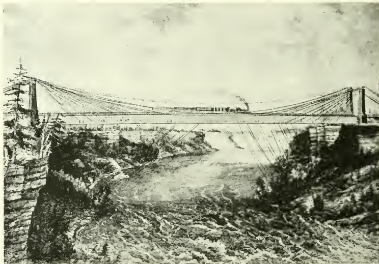
THE GRAND TRUNK RAILWAY SUSPENSION BRIDGE.
